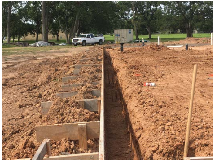
2. Excavation of grade beams for slab on grade
