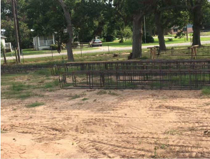
1. Site fabrication of reinforcing steel
